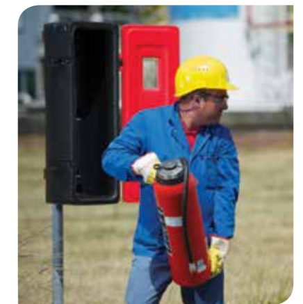
Small fire extinguishers in the neighborhood of peroxide stores
