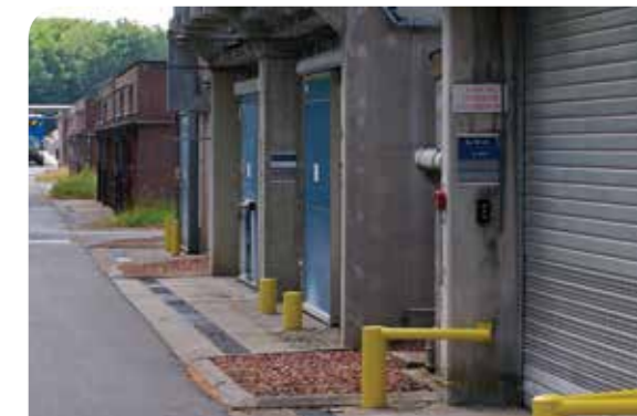
Organic peroxide storage rooms
